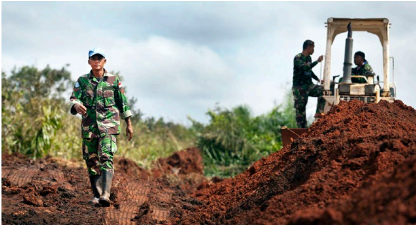
Indonesian Engineer Company during road construction
