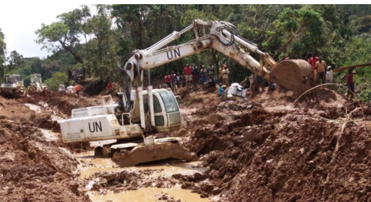
rehabilitation of Dungu-Duru road
