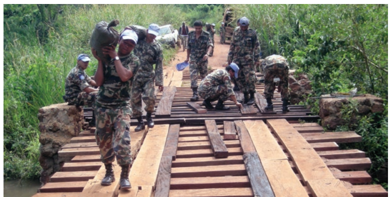
Nepalese Engineers Company during bridge maintenance
