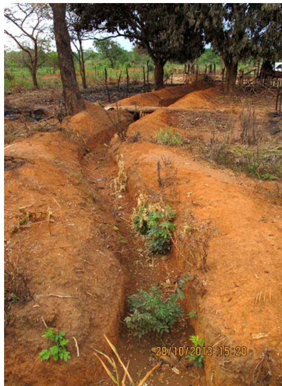
Trench dug around the perimeter of the FARDC base.
