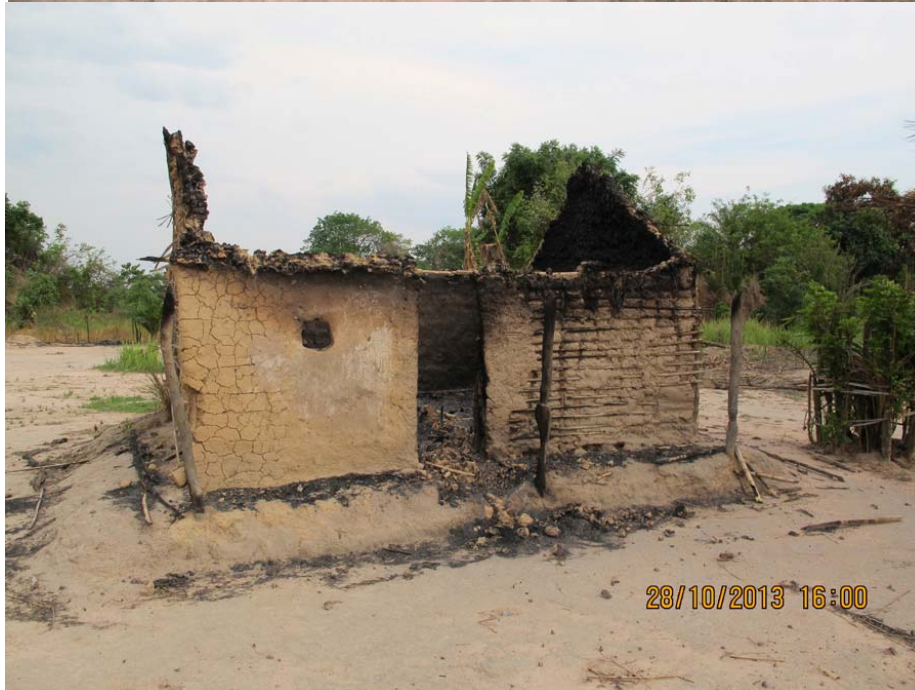
Structures in Katendeji village, which were burned by Kata Katanga.
